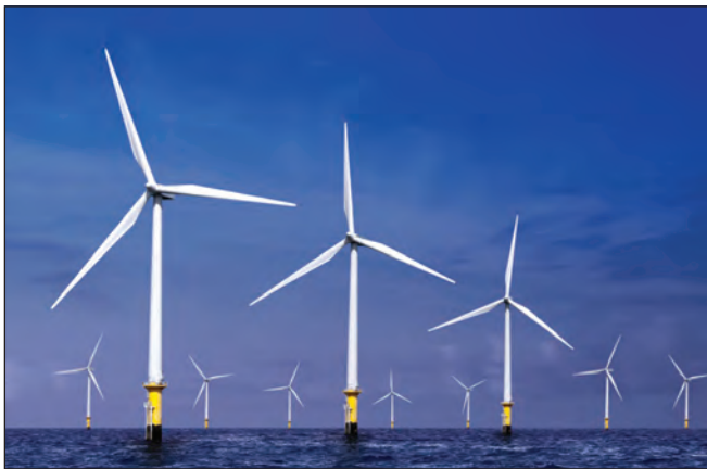
Xylan industrial coatings drive down "life-operating" costs.
