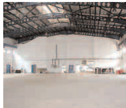
A view of some of the 4,600 square meters of space that will be designed to the highest, most efficient manufacturing standards.
