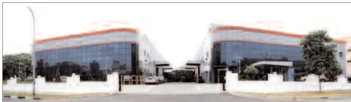
A wide-angle view of the new Singapore facility prior to the extensive renovations that Whitford is making to both buildings, which include covering the area between the two to unite them.
